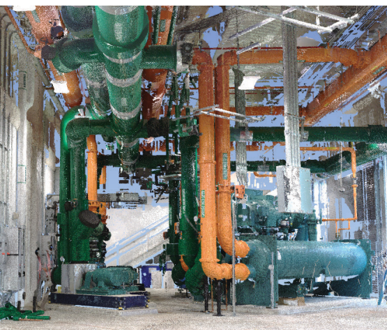
Mechanical Room Scan of Existing Plan
